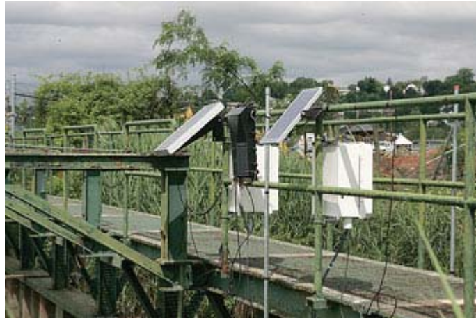
Figure 23 Tide Gate at West Riser with Water level Sensor and Data Transmission Hub
